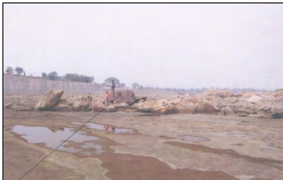
Existing Hard Rock to be cleared in Spill Channel
